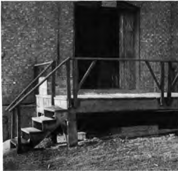
Fig. 1. Removable Railing at Loading Platform.*
